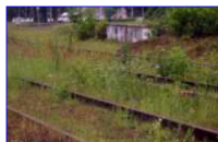
The former Ramp, left Part
